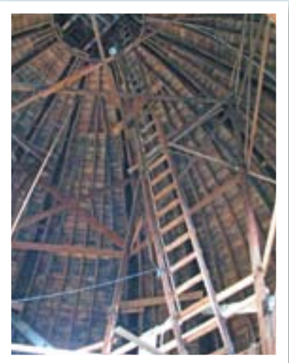
Picture of the dome interior with the ladder to the top.
